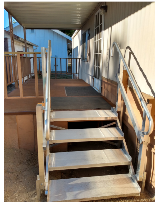
Photo: La Casita new stairway and landing. Photo by Michele Jimenez-Holtz
